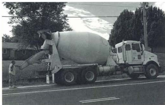
Above: A construction worker takes a break from the late summer heat. The road construction took several months to complete. Photo by Linda Shireman
