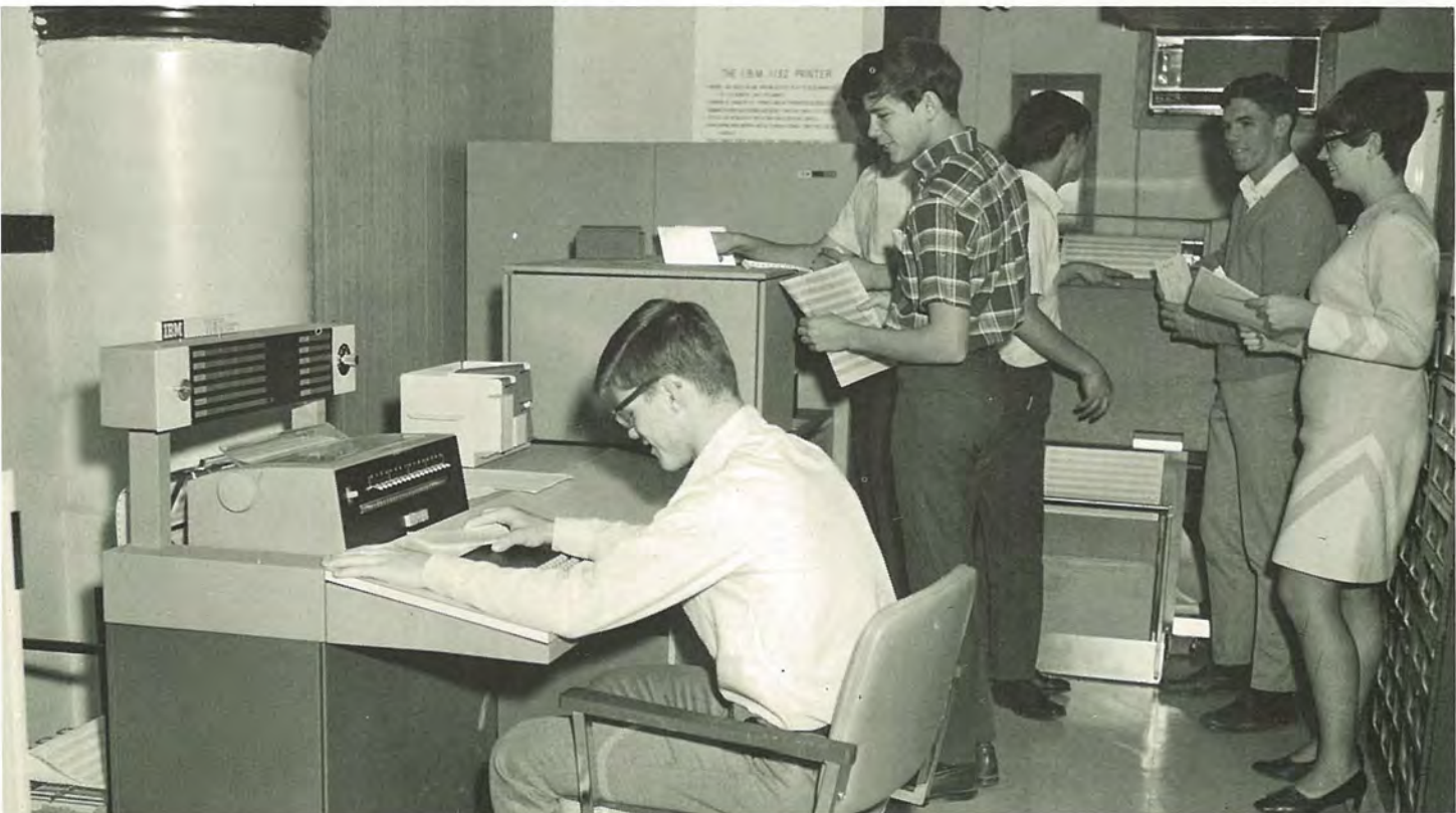
The Computer Center in operation with IBM 1130 equipment.
