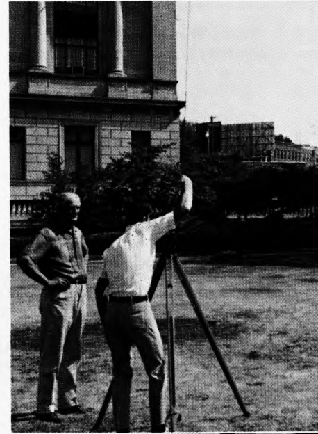
On-the-site use of the transit adds reality to the student's work in such courses as surveying and slide rule.
