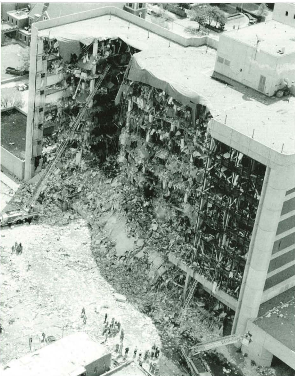
The Alfred Murrah Federal Building in downtown Oklahoma City sits in ruin after the explosion on April 19. After recovery efforts ceased, the building was determined unsafe and was imploded.
