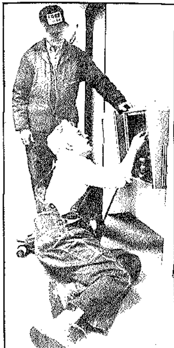
1:30 p.m.—Leonard Elliott (sitting) and O.B. Vincent repair a broken water fountain in the SSC Building. Photo by Todd Scrivers.
