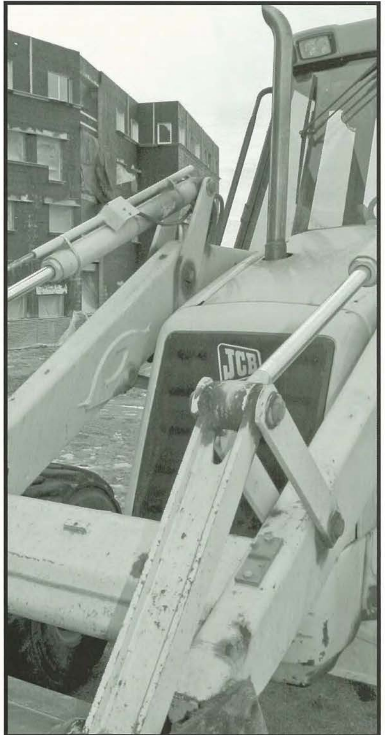
Construction machines are a constant reminder to students that construction is almost finished. Students waited in anticipation for the finishing touches of the new residence halls.
